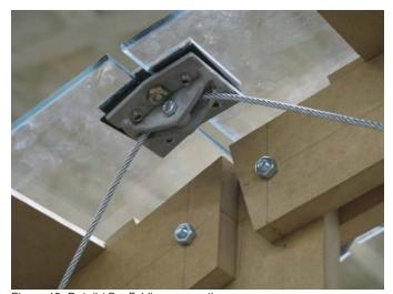
Figure 13: Detail / Scaffolding connection
