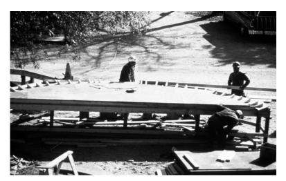
5. Carpenters preparing formwork for cycloid shells. Forth Worth, 1969.
