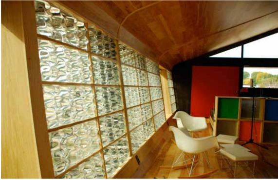
the elevated floor to circulate upward through a gap between exterior-mounted, double-paned Low-Emittance (Low-E) glass and the interior-mounted water wall. This flow of air over the water wall cools the individual plastic containers, which, in turn, siphon heat from the interior space. The rising air then continues into a tapering gap (Venturi effect) under the photovoltaic array, thus cooling the underside of the roof panels.
