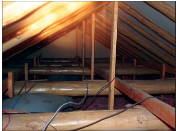
FIG. R2.7: Concealed rustic pitched ceiling above the suspended ceiling (accessed through a vent), 2007.
