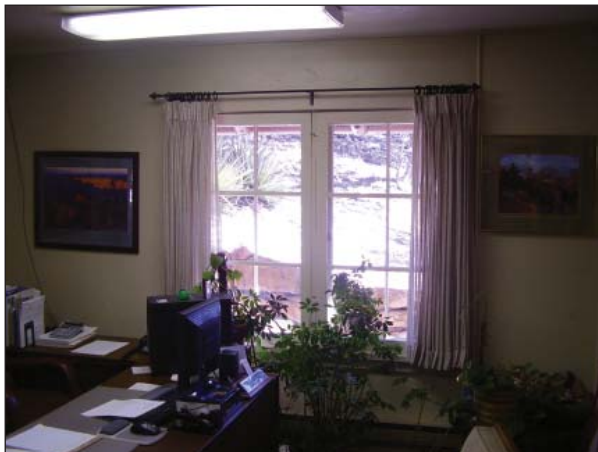
FIG. R5.2: View of Room Five facing east showing the double six-lite wood casement windows and concealed picture rail, 2007.
