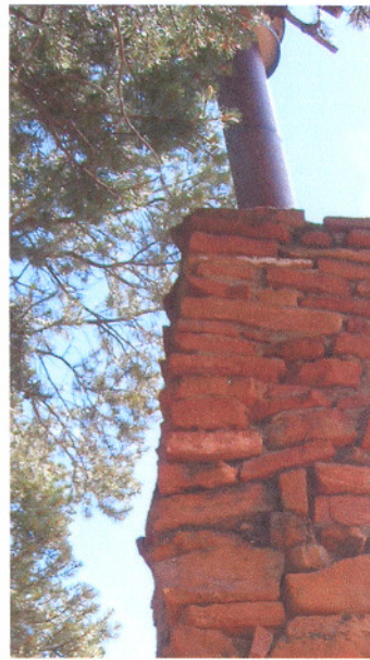
2. Skewed Metal Flue Chimney
