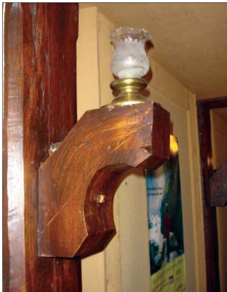
FIG. R18.10: Incandescent light fixture on wood post corbel, 2007.
