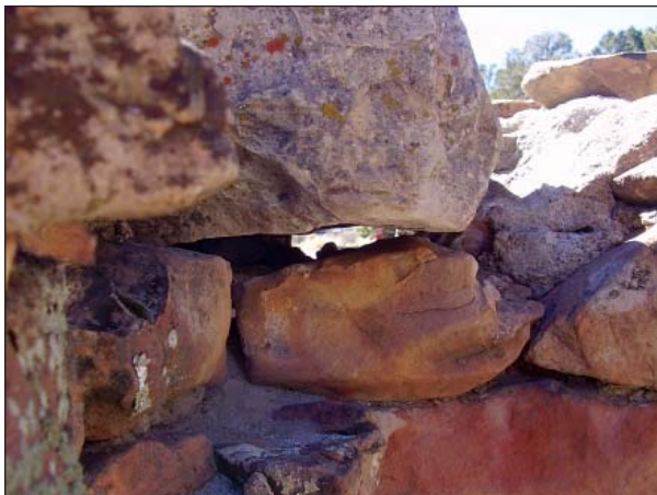
FIG. E17: Gaps in the southwest corner of the patio stone support, 2007.
