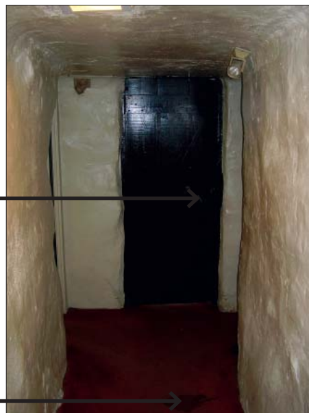
FIG. LH7: View of the dimly-lit hallway facing south showing the historic wood door to Room Eighteen and floor deflection. Note locking mechanism on the hallway-side of the door and carpet stain at arrows, 2007.
