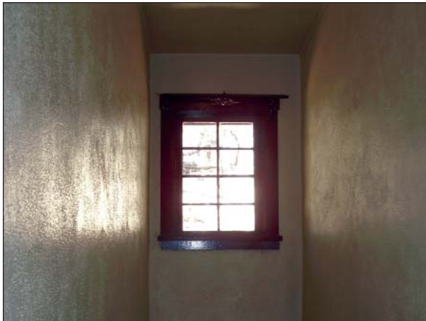
FIG. LH4: Eight-lite wood casement window on the north stairwell wall, 2007.
