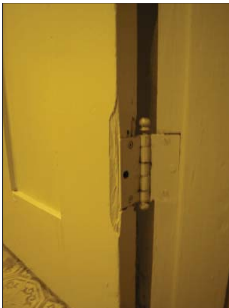
FIG. R13.6: Split door stile. Note coloration in photograph is due to flash photography, not actual appearance, 2008.
