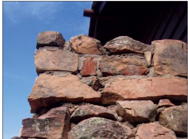
FIG. E20: Lichen on the stone on the east wall, 2007.
