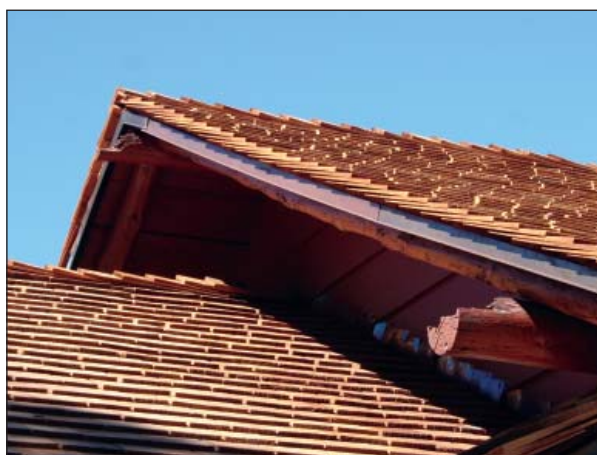
FIG. E6: Decayed outriggers on the south wall, 2007.
