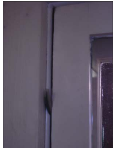
FIG. R5.7: Damaged weatherstripping on the north window, 2007.
