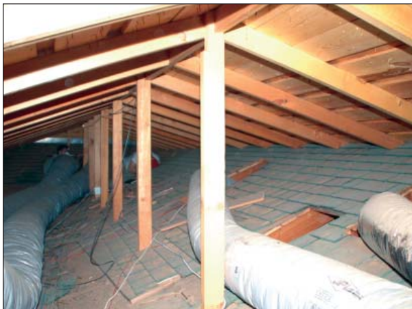
FIG. E9: View into the attic where a roof was superimposed over an earlier pitched roof showing the web of flexible duct and potentially hazardous asphalt shingles on the earlier roof, 2007.
