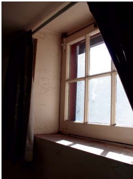
FIG. R17.2: Six-lite wood hopper window on the west wall of Room Seventeen, 2007.
