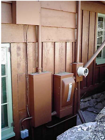
Figure 6: Electrical service entrance on exterior east wall
