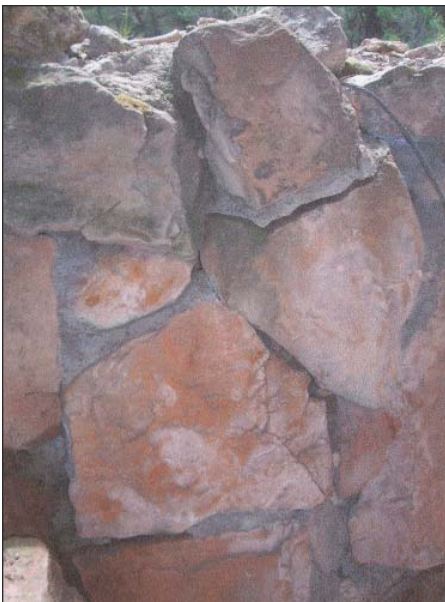
FIG. S19: Loose stone and cracked mortar in buckling east stone retaining wall, 2007.
