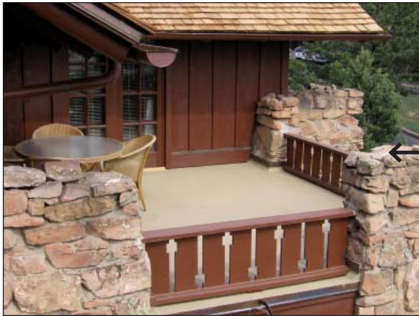
FIG. E15: View of the patio facing southeast showing the structural stone corners, wood railing and liquid-applied, waterproofing membrane flooring. Note birdbath location at arrow and low railing height, 2007.
