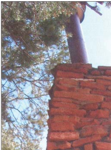
FIG. E21: Skewed metal flue on the Room Two chimney. Note dangerous proximity of tree, 2007.
