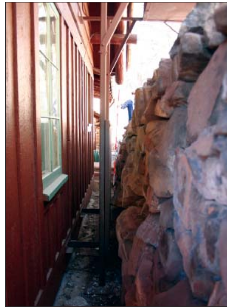
FIG. S10: Buckled stone retaining wall on the north side of the building, 2007.
