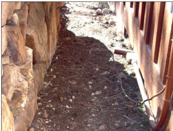
FIG. S15: Debris-filled walkway near the northeast retaining wall that directs water toward the foundation, 2007.
