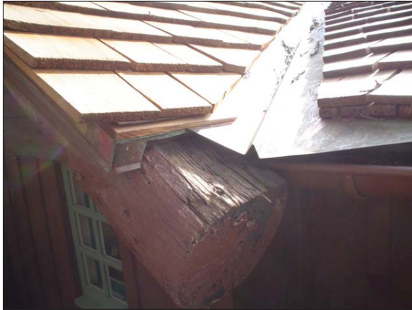
FIG. E7: Water directed onto a rafter from the roof valley on the north wall, 2008.
