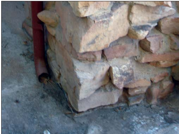
FIG. E13: Downspout on the northwest corner of the building that drains water onto the patio floor and toward the building foundation, 2007.
