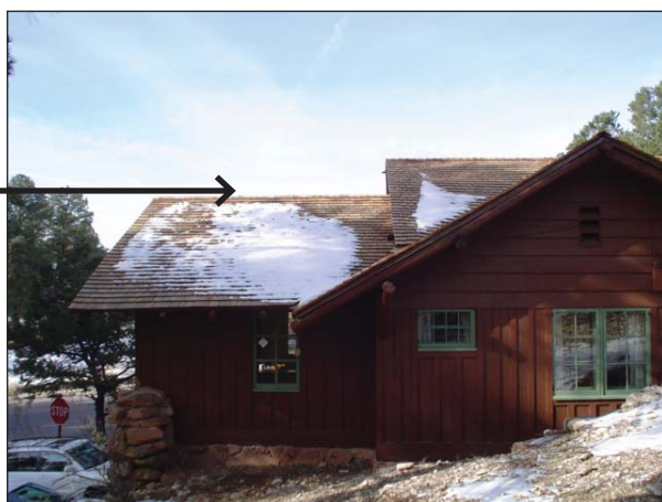
FIG. E5: East wall showing the deflected roof over Room Eight at arrow, 2008.
