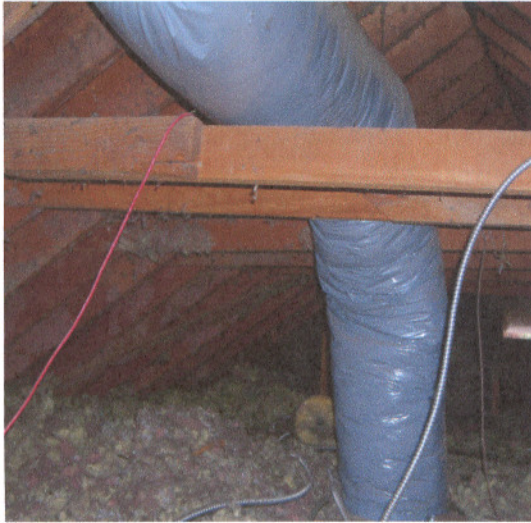
13. Split and partially repaired collar tie
