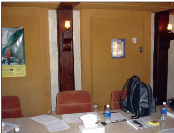
FIG. R18.6: View facing north showing the modern tack surfaces between the original wood posts, 2007.
