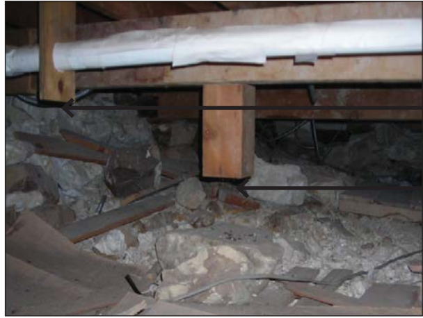
FIG. LH11: Displaced stones and missing supports under posts in crawlspace at arrows, 2007.
