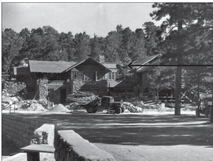
FIG. CD5: South wall of the addition under construction. Note the roof between the two gables at arrow which had a railing and was since covered by a superstructural roof, 1931 (Source: GRCA Museum Collection, Photograph 151).
