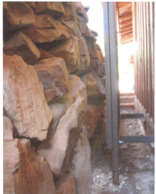
6. Stone wall bulging into wood board
