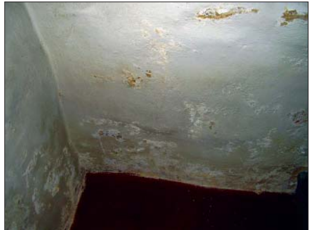
FIG. LH5: Water damage on the exposed stone walls at the northwest corner of the stairwell, 2007.
