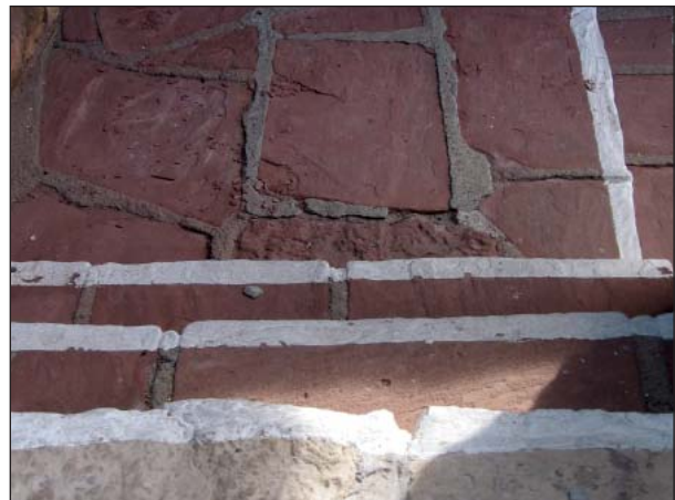
FIG. S12: Uneven pathway and steps due to differential weathering of materials, 2007.
