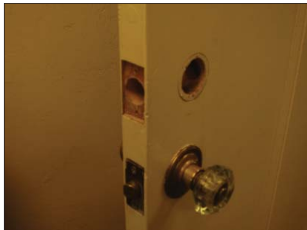
FIG. R4.3: Door missing deadbolt, 2007.
