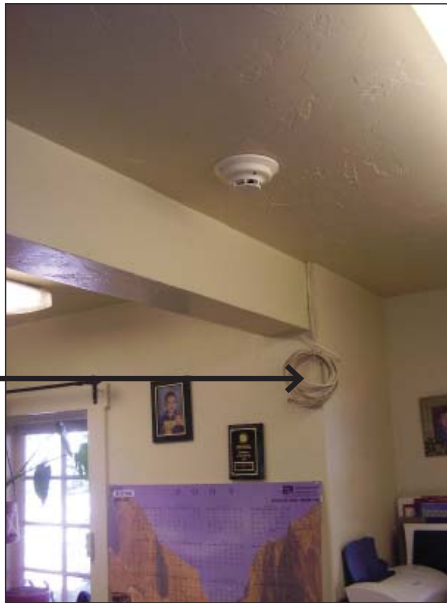
FIG. R4.4: View facing north showing the structural remnant of the removed partition wall. Note exposed wiring at arrow, 2007.
