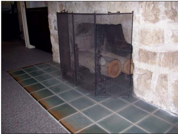
FIG. R11.4: Fireplace hearth and tile. Note adjacent carpet conceals the historic wood flooring, 2007.
