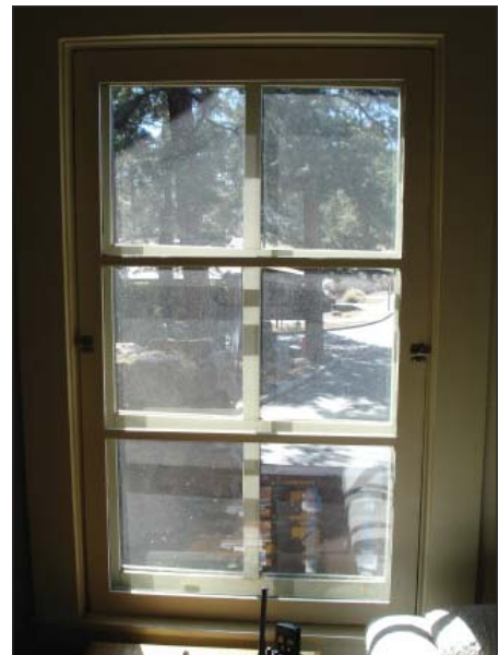
FIG. R11.7: Six-lite wood casement window on the south wall, 2007.
