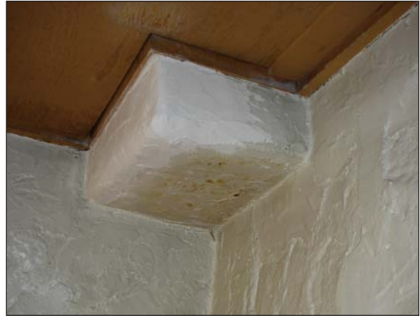
FIG. R18.9: Drop chase located in the northwest corner of Room Eighteen, 2007.
