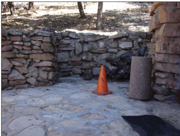
FIG. S11: Uneven paving near the entrance to Room One due to differential weathering of materials. Note the north stone retaining wall in the background, 2007.
