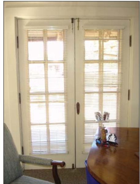
FIG. R11.5: Double eight-lite wood doors to the upper level patio on the west wall, 2007.
