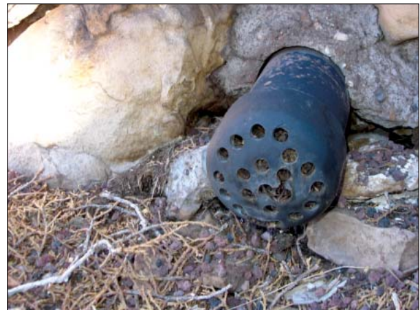
FIG. S16: Debris-filled drainage pipe on the south stone patio wall, 2007.
