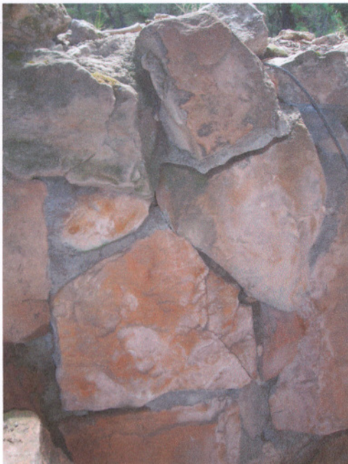
7. Bulge in wall – mortar separating from stone
