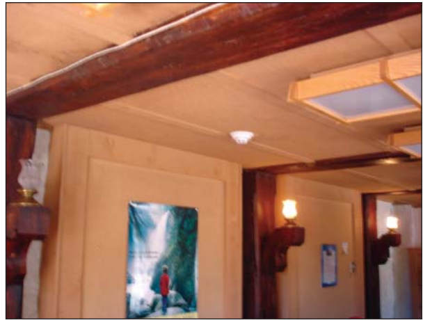
FIG. R18.5: Modern suspended plywood ceiling with east-west battens situated between the original north-south wood beams, 2007.
