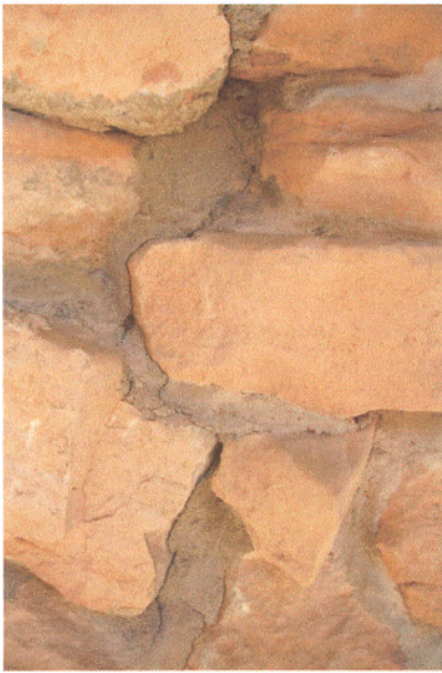
1. Minor cracks in stone masonry chimney
