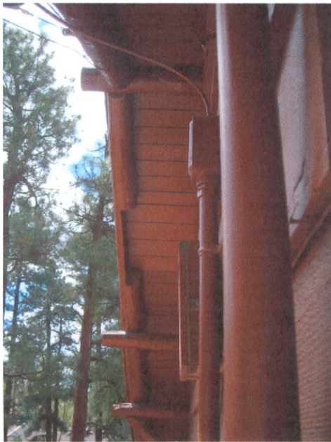
9. Missing portion of fascia beam
