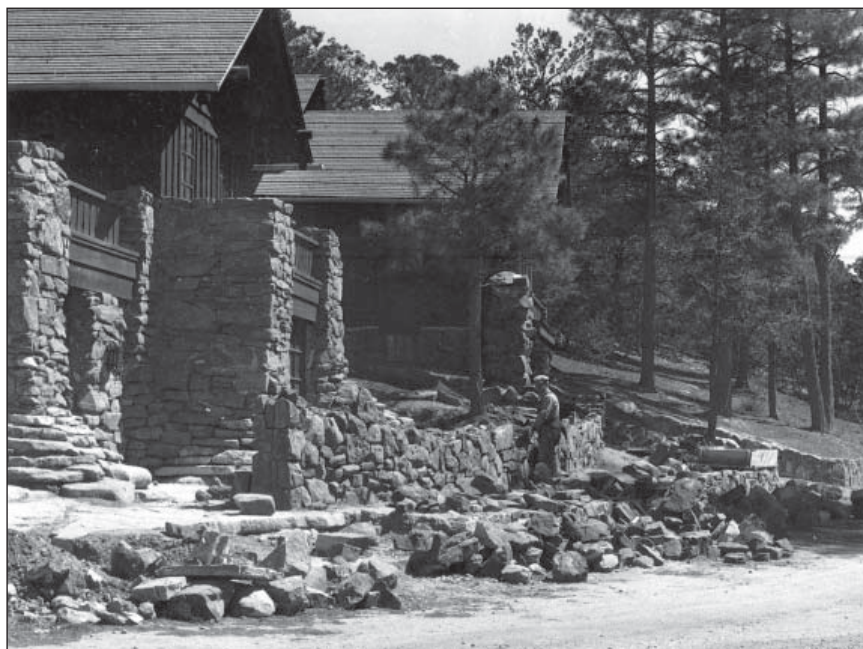
FIG. CD7: Patio wall under construction in front of the First Administration Building, 1932 (Source: GRCA Museum Collection, Photograph 148).
