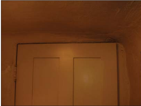
FIG. R13.4: Plastered door frame. Note coloration in photograph is due to flash photography, not actual appearance, 2007.
