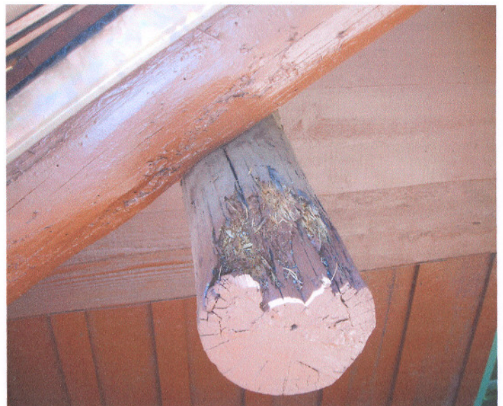
8. Weather deteriorated exposed ends of outlookers
