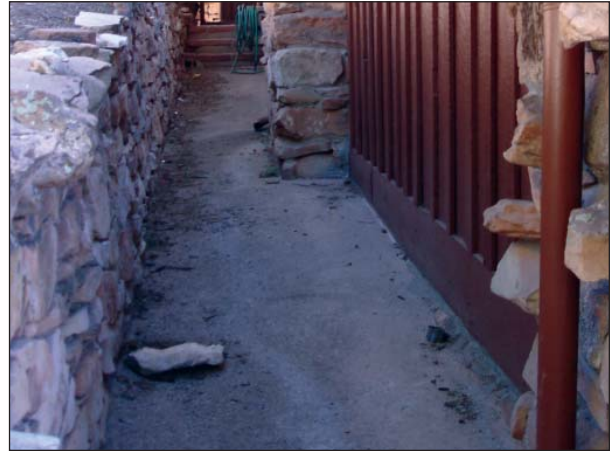
FIG. S14: View facing west showing the concrete walkway that directs water toward the building, 2007.
