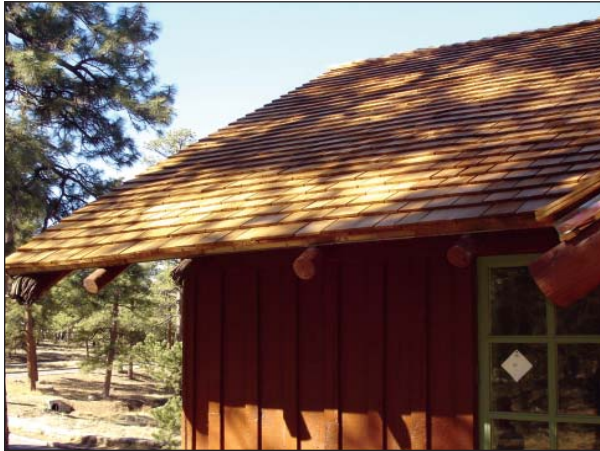
FIG. E11: Missing gutter on the south side of the east wall, 2007.
