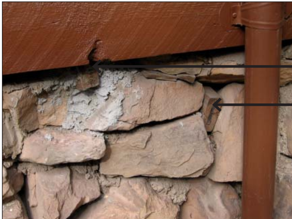
FIG. E19: Wood in-fill in the stone wall on the south wall at arrows, 2007.
