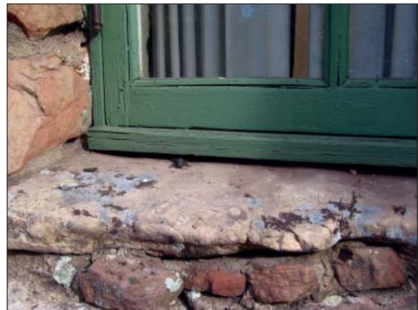
FIG. E26: Gap between the window and stonework on the south wall, 2007.
