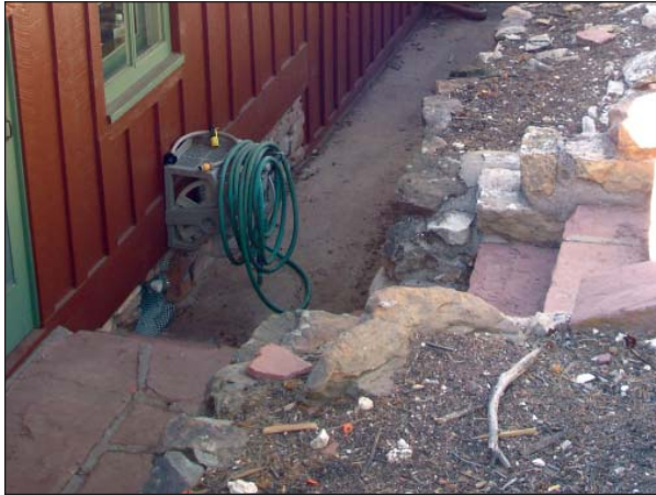
FIG. S13: View of the north stair showing site slope that directs water toward the north side of the building, 2007.
