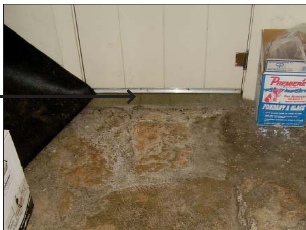
FIG. R1.4: Original stone floor cracking at joints. Note cracked threshold at arrow, 2007.
