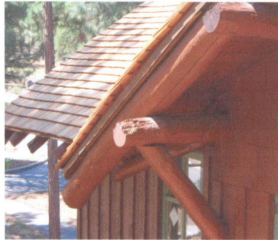
10. Braced and sagging gable end
