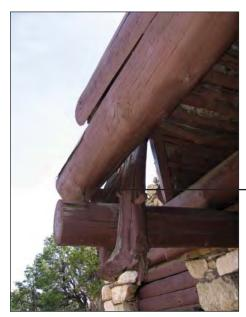
FIG. E25: Displaced porch beam at arrow, 2007.
