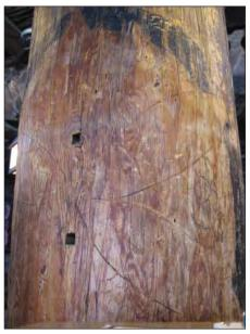
FIG. GR14: Post showing etched lines, faded paint and holes where candelabra was once mounted, 2007.
