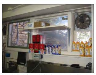
FIG. K12: West windows showing window film, exhaust fan, storage shelf and blocked daylight, 2007.
