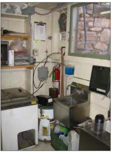
FIG. K9: Southwest corner of the Kitchen showing the freezer at left, hot water heater at center, and sink at right. Note the exhaust fan in the window in the corner and wiring over the fire extinguisher, 2007.
