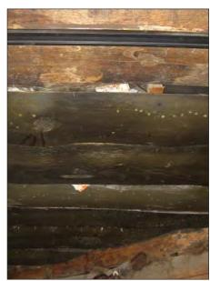
FIG. GR8: Modern log slab ceiling at the entrance showing the debris collected by rodents, 2007.
