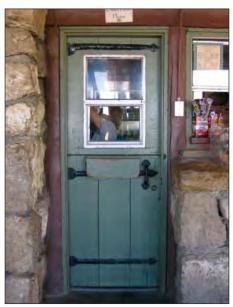
FIG. E40: Kitchen Dutch door with modern alterations including double-hung aluminum frame window and fold down shelf, 2007.
