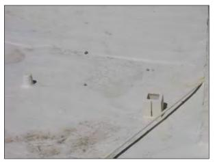
FIG. E33: View of the roof showing the concrete block and unsecured propane pipe, 2007.
