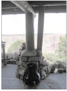
FIG. E27: Downspout (right of log post) encased in a wood box which is presumed to lead to a cistern beneath the porch floor at left, 2007.
