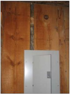
FIG. SR18: Missing batten in the storage closet, 2007.
