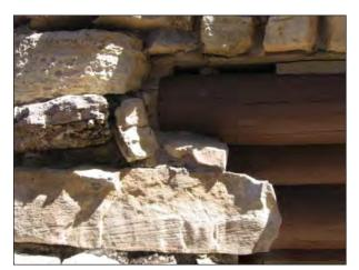
FIG. E15: Gap between a lintel and stone allowing rodent access to the building interior, 2007.
