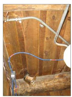
FIG. H4: Ceiling treatment on the south side of the Hall. Notice water damage behind light fixture at right, 2007.
