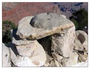
FIG. E13: Mortar applied on top of the roof lookout, 2007.
