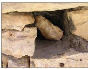
FIG. E14: Missing stone on the west elevation allowing rodent access to the building interior, 2007.
