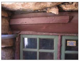
FIG. E58: Damaged  $2\times 4$  applied on the lintel above the Office window on the west elevation. Note electrical conduit entering the building through the window trim at left, 2007.
