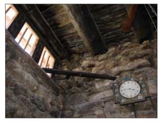
FIG. GR7: View of the southeast corner of the Great Room showing the stone walls, wood ceiling and windows, painted clock and steel c-channel for the removed propane heater. Note conduit in corner, 2007.
