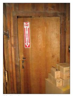
FIG. SR7: Closet door on the south side of the west wall currently oriented with the iron strap hinges facing the closet interior, 2007.
