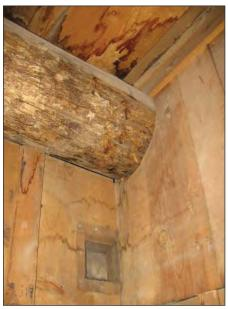
FIG. SR13: Water damage on the closet ceiling and a screen over a hole in the wall, 2007.
