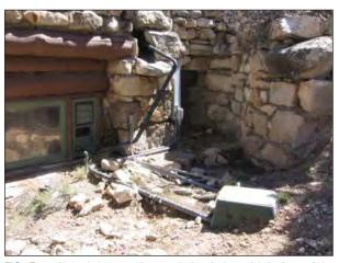
FIG. E56: Unburied water pipes and electrical conduit in front of the west elevation. Note grey water pumps upward in pipe situated on the drainage, 2007.
