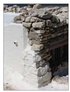
FIG. E32: Roofing material and excessive mortar applied to the stone at southeast corner of the building, 2007.
