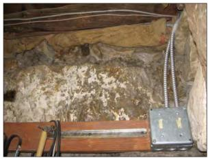
FIG. H6: North wall showing conduit. Note burlap in-fill between wall and ceiling, 2007.
