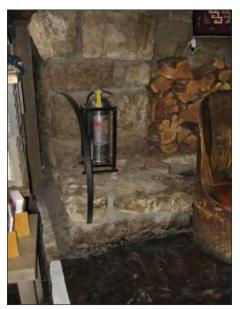
FIG. GR11: Built-in bench showing the iron firewood holder and incompatible mortar, 2007.
