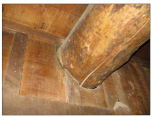
FIG. SR14: Gap between a ceiling beam and wall, 2007.
