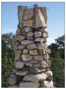
FIG. E10: Missing stones and mortar creating holes in the in Secondary Room chimney. Note unsecured wire mesh, 2007.
