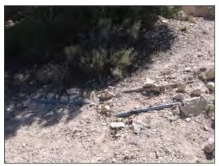
FIG. S21: Exposed water pipes, 2007.
