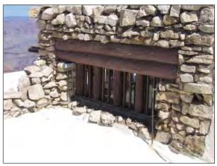
FIG. E53: West clerestory showing the electrical conduit through the window frame at bottom right, and propane conduit through mortar adjacent to window frame at center, 2007.
