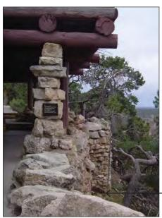
FIG. E16: View of the Hermit's Rest porch facing west. Note displaced stones at arrow, 2006.
