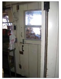
FIG. K3: Dutch door on the north wall showing the modern aluminum window, 2007.
