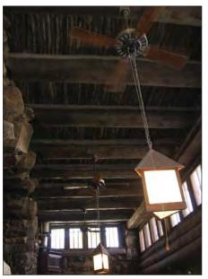
FIG. GR5: Great Room ceiling showing log beams, latilla, clerestory windows, propane heater, modern ceiling fans and modern light fixtures, 2007.
