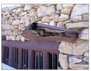
FIG. E36: Decayed vigas covered with sheet metal at the north elevation clerestory, 2007.
