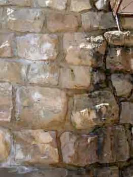
Figure 11 & Figure 12 - Efflorescence and erosion caused by poor drainage.
