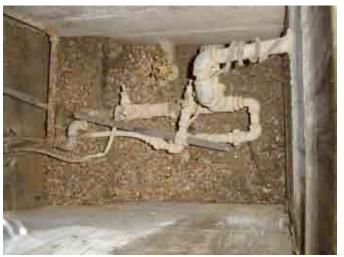
Figure 22 & Figure 23 - Manhole cover in Repair Shop and old water supply and air piping system, within the manhole.
