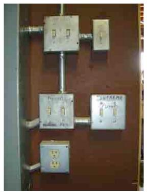
Figure 30 & Figure 31 – Original electrical outlet in Repair Shop using conduit embedded in concrete slab (left) and non-functioning switch boxes in Utility Room (right).
