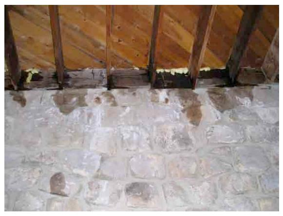
Figure 13 - Water leakage in the interior of the Utility Room between the stone wall and roof plane caused by poor water drainage and inappropriate flashing at connection between stone wall and built-up roofing membrane.
