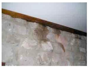
Figure 54 & Figure 55 - Wooden toilet stall partitions (left) and water damage from poor connection between stone wall and roof in Women's Restroom (right).
