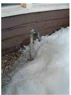
Figure 26 - Exterior water spigot, no longer functional.
