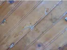
Figure 62 & Figure 63 - Water damage to paneled ceiling and wood trim.
