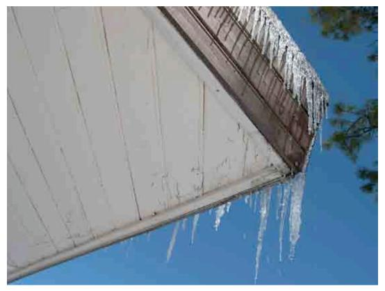
Figure 9 - Water drainage occurring at the fascia of the Pump Canopy causing damage to the wood fascia members due to an unintentional drainage system.
