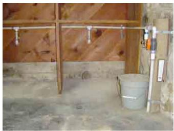
Figure 24 & Figure 25 - Current PVC water supply system as it enters the building in the Utility Room (left) and is distributed to the restrooms (right).
