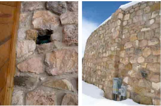
Figure 36 & Figure 37 - Location of flue hole on the interior of the Repair Shop (left) and the protruding chimney form on the exterior of the west wall (right).
