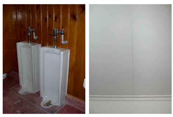
Figure 59 & Figure 60 - Original urinals showing integrated concrete floor slab and base molding (left) and crack in ceiling plasterboard, visible in both Men's and Women's Restrooms (right).
