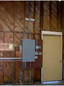
Figure 28 & Figure 29 - Upgraded electrical system enters building through stone wall (left) to the panel distribution box in the Utility Room (right).
