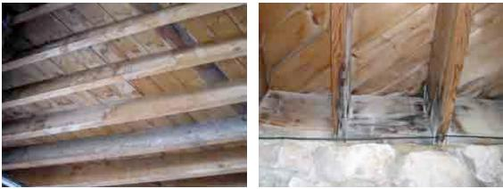
Figure 19 & Figure 20 - Areas of water damage to roof joists in Repair Shop (left) and Utility Room (right).
