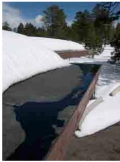
Figure 5 & Figure 6 - Water ponding on the roof causing damage to the stone wall and at the roof's edge adjacent to the fascia.
