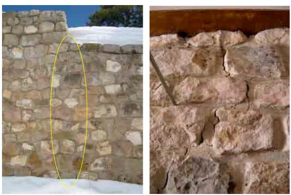
Figure 17 & Figure 18 - Large crack in rear stone wall, exterior (left) and interior (right, in Women's Restroom).
