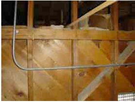
Figure 75 & Figure 76 - West stone wall showing the water stains at the connection between the stone wall and roof joist, the dripping foam used to unsuccessfully seal the joint (left) and the east exposed wood frame wall with the intersticiary space above (right).
