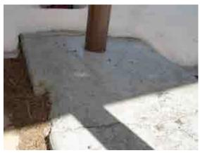
Figure 15 & Figure 16 - Areas of concrete slab cracking and minor loss around the building exterior.
