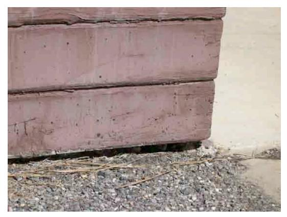
Figure 10 - Undercutting at the SE corner of the Sales Office, caused by poor site drainage.
