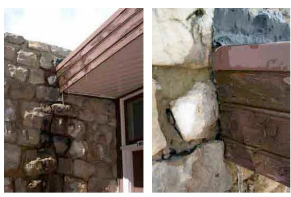
Figure 7 & Figure 8 - Poor drainage at the southwest corner of the building showing water damage to the stone wall and the fascia.
