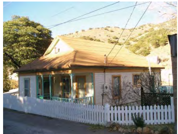
Fig. 15.20 – 519 O'Hare Ave, Higgins Hill; an example of a gable-on-bip roof type with a front porch integrated within the roof form. Courtesy of R. Brooks Jeffery
