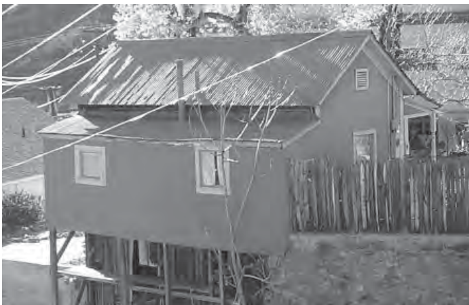
Fig. 3.6 – Hall-and-parlor side gable house type with a drop shed porch and rear addition, School Hill, Bisbee. Courtesy of R. Brooks Jeffery
