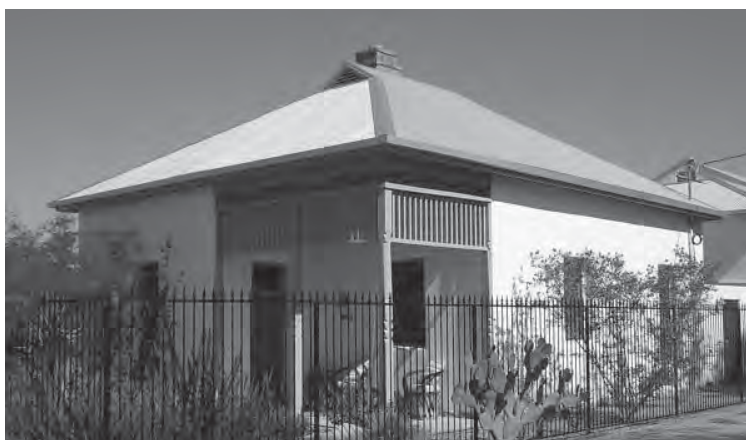
Fig. 5.7 – Gable-on-bip pyramidal cottage house type with a louvered roof vent and entry porch carved out of the square plan, Barrio Viejo, Tucson. Courtesy of R. Brooks Jeffery
