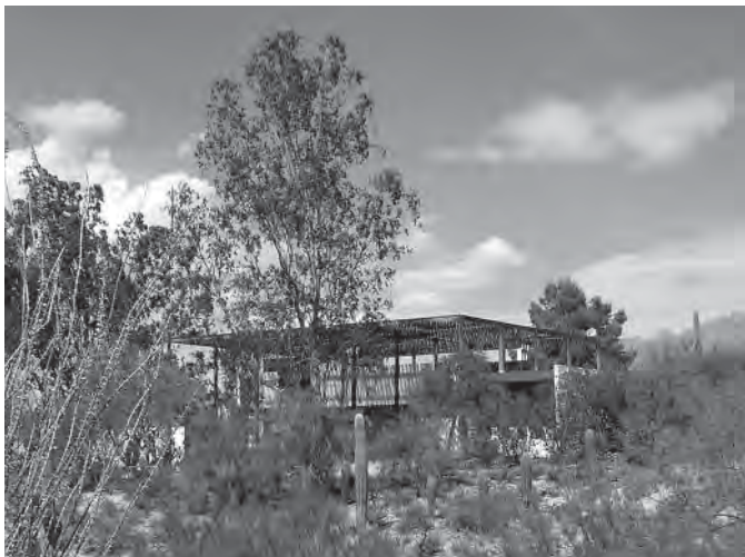
Fig. 7.2 – Ramada House, Tucson by Judith Chafee, 1975 uses a large ramada structure to provide a blanket of shade over the body of the house. Courtesy of Michael Lovato
