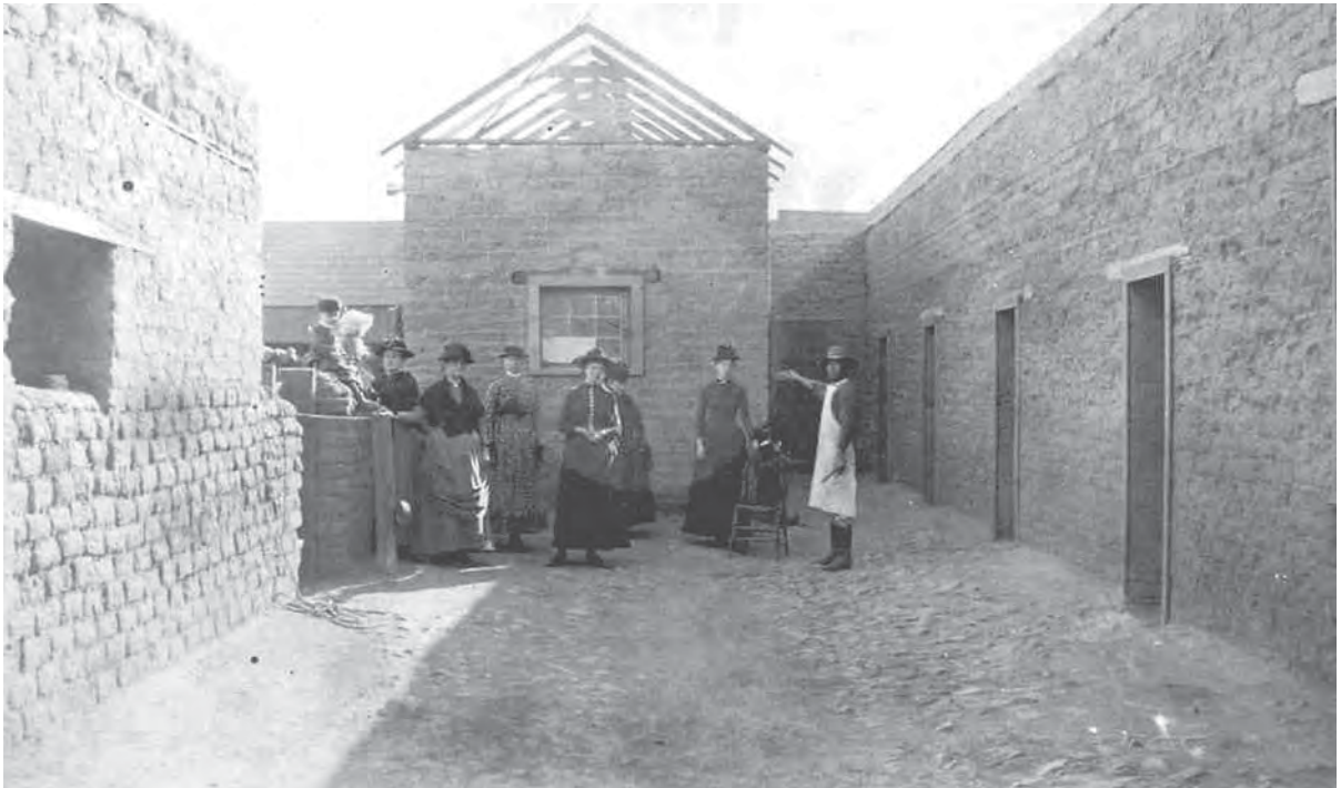
Fig. 12.5 – Ladies and cook in the patio, ca. 1885. A pitched roof is being constructed over the cook's quarters (Rooms 16 and 18). It is interesting to note that nearly all of the doorways on the right were later changed to windows, as the orientation and use of the building changed. Courtesy of Empire Ranch Foundation/Laura (Dusty) Vail Ingram/Bureau of Land Management (Image # A300-062)
